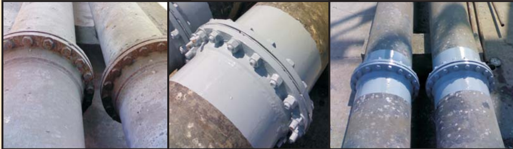
Galvanic and Saline Corrosion Protection of Pipeline Flanges
