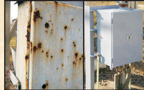
Corrosion Protection of substation Marshalling Boxes
