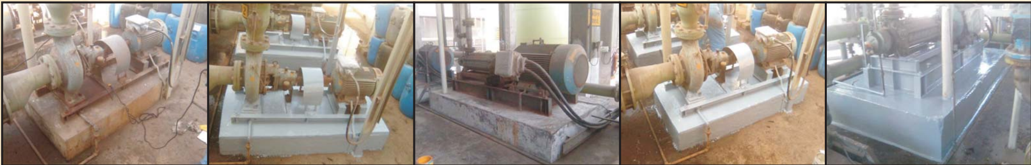
Corrosion Protection of Water Pumps, Motors, Foundations from water spills
